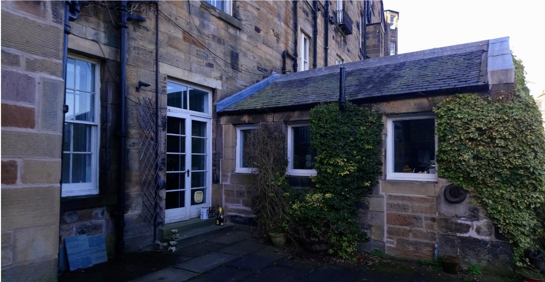
View 2 External view from terrace.
