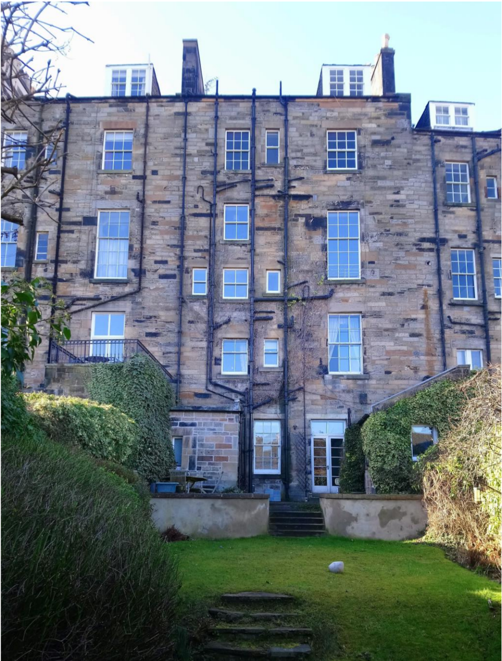
View 3 Full rear elevation from garden
