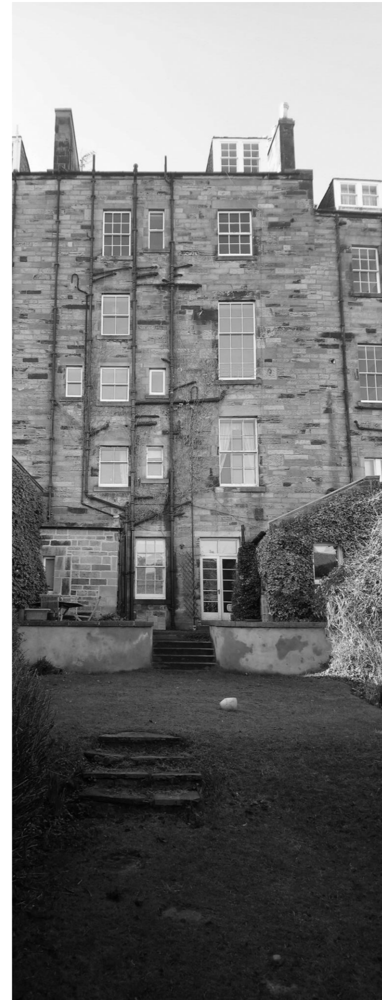
13 Clarendon Crescent: View from rear garden.
